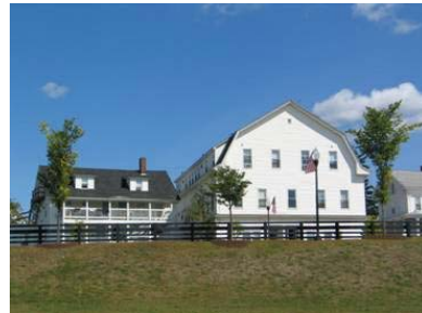
14 affordable housing units in a multi-family in Laconia
