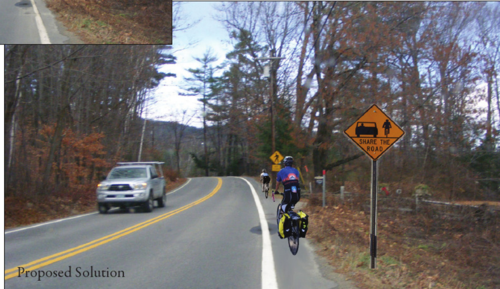
Conceptual rendering of a lane width modification along NH Route 113 in Holderness. Existing 11½ - 12 foot lane is shown above. Proposed improvement with 10½ - 11 foot lanes using existing pavement is shown below, with added ‘Share the Road’ signage.
